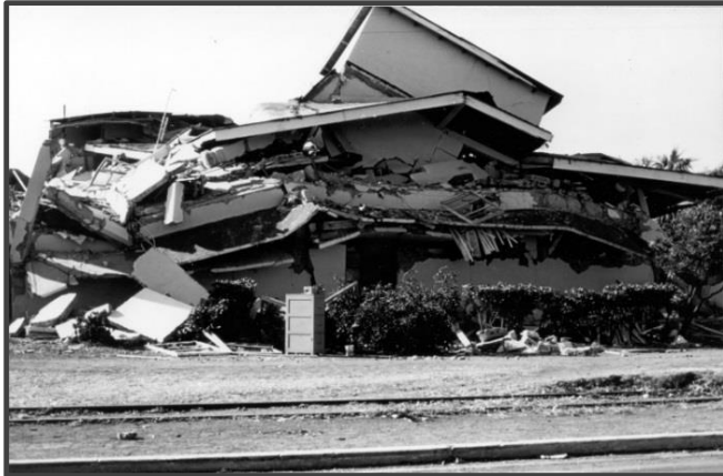
Nicaragua Earthquakes December 1972, Managua. Collapsed Three-story reinforced concrete Customs House office building (Source: USGS)
